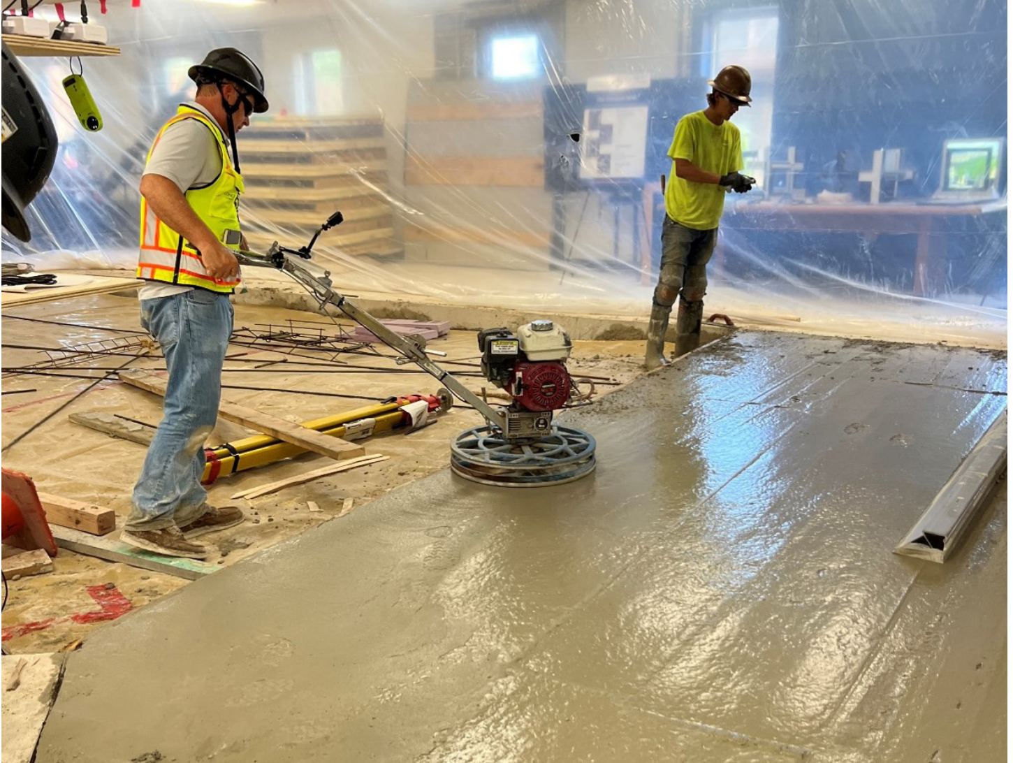
Placement of Mixture #3 showing the gas-powered walk-behind trowel finisher in use
