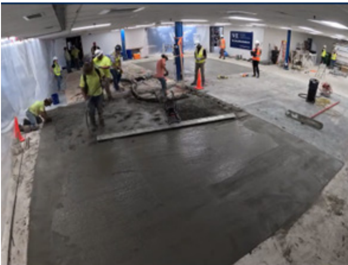
Placement of Mixture #2 showing the finishing sequencing
