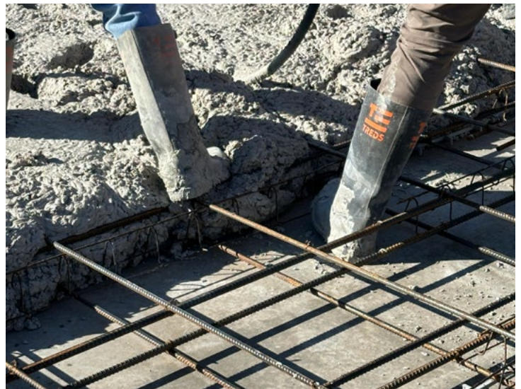
Placing novel 1157 mix for Panel 3.
