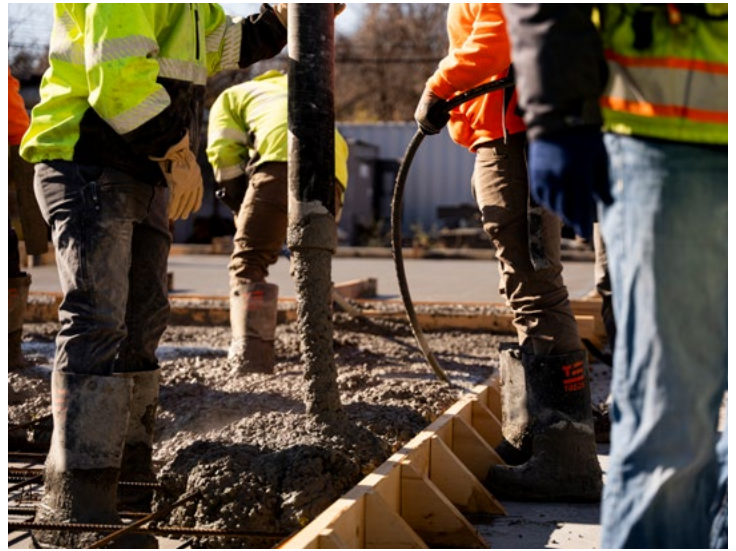
Placing crew working on Panel 2.
