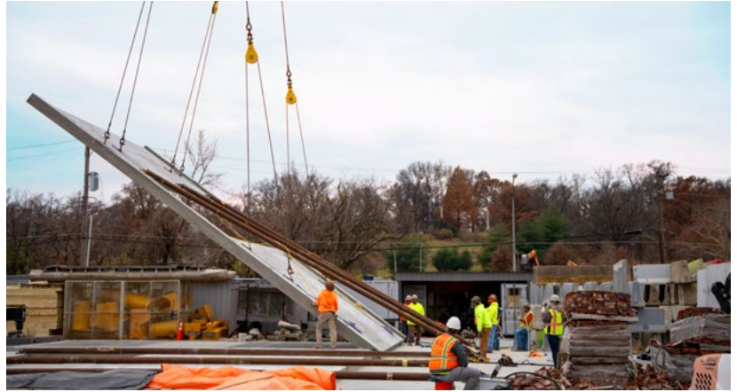
Erection of Panel 1 and 2 occurred on day 3.
